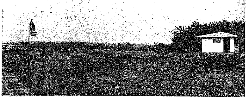
Fig. 1. The new seismograph station at Hilo, Hawaii.
