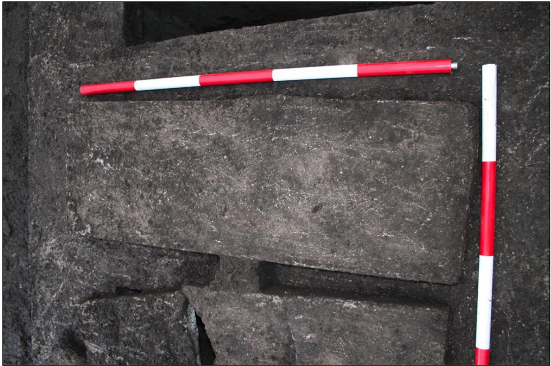
Plate 2.4: Concrete lid consistent with original concrete structure
