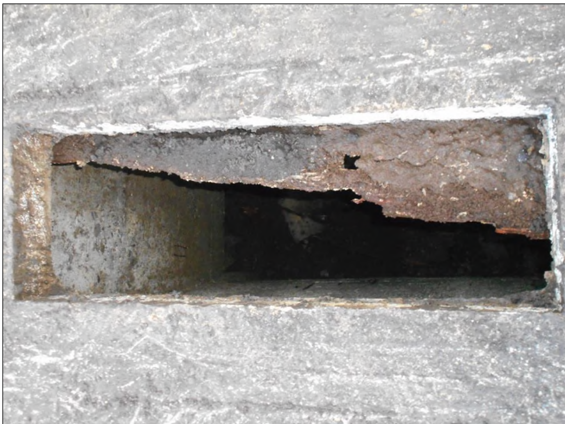
Plate 2.3: Timber formwork in situ at C.46/47/62/63
