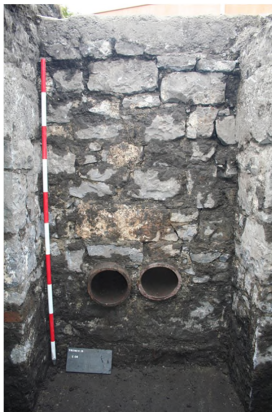
Plate 2.7: North wall of tank with inlet pipes
