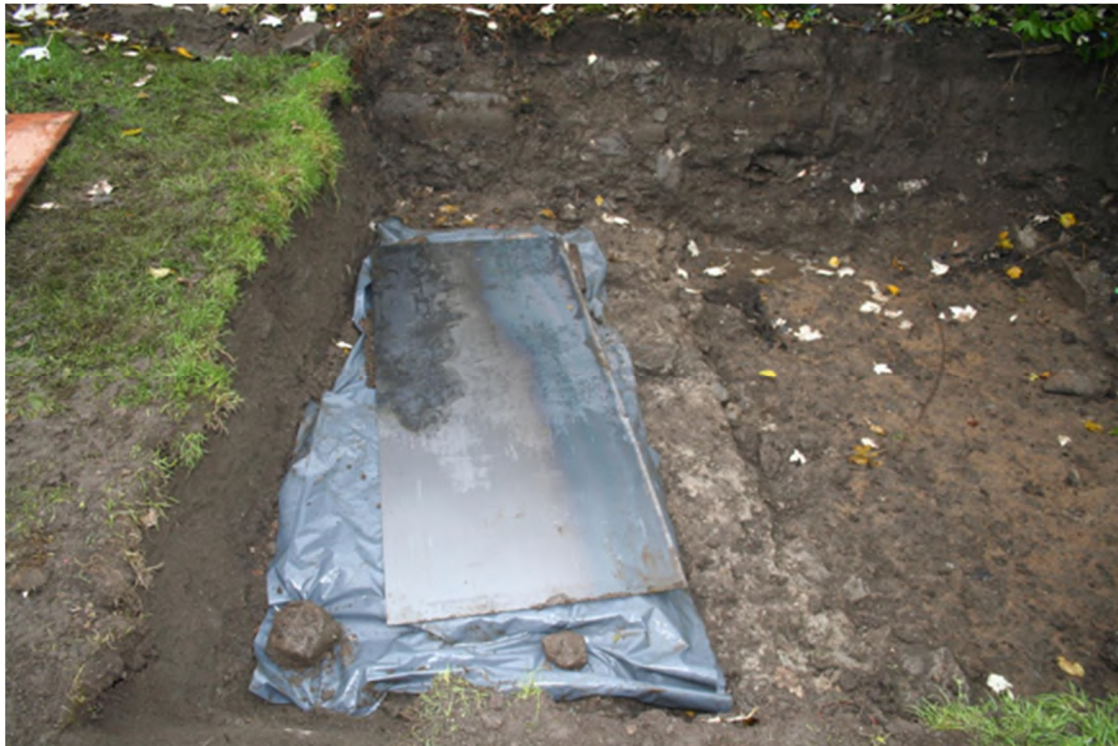
Plate 6.1: Sealing of chambers prior to backfilling site
